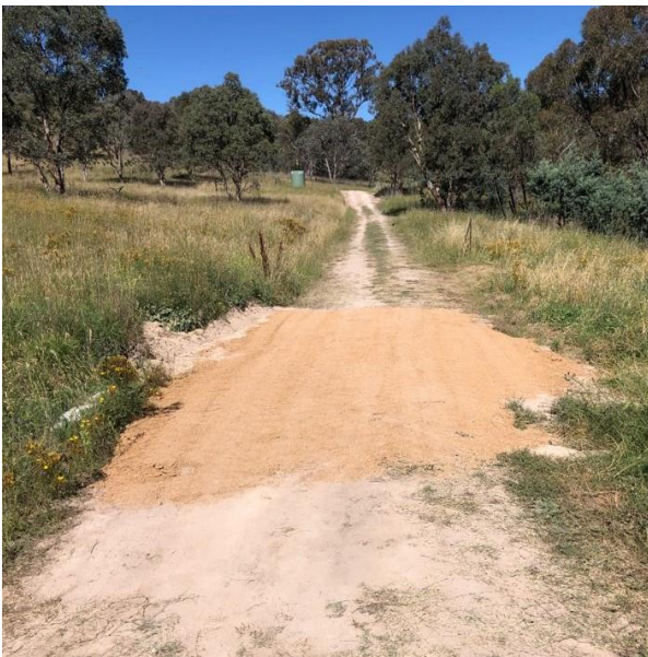
Newly repaired BNT
